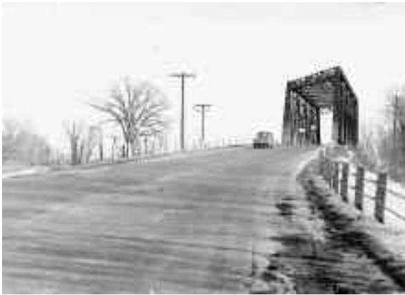
The “Wart,” East Victor Bridge, 1922 (seen here in 1964).
