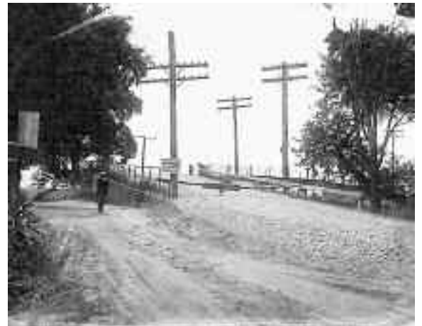
The original Lehigh Valley Crossing on left, new construction on right, c. 1921.
