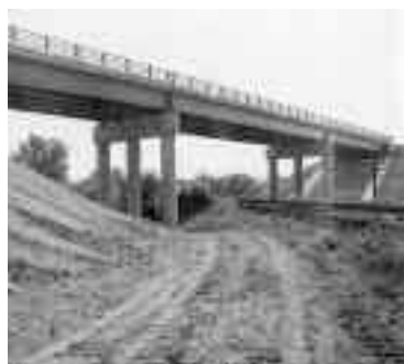
September 8, 1965 East Victor Overhead Bridge.
