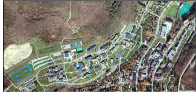
Aerial Photographs available through Pictometry Technology Showing Village of Alfred
