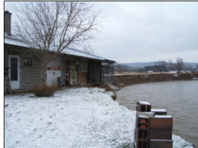
Washouts Along Local Rivers & Streams
