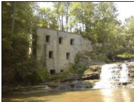
Historic Electric Plant at Wiscoy Falls
